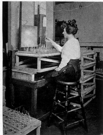
Moorhead Laboratories. Inspecting for defects after sealing.
